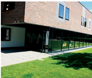
Kings Road Entrance (taxi drop-off/collection point)
